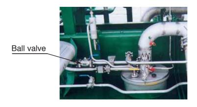
Mild steel valves are delivered with primer only. During replacement a proper coating must be applied to the valves, and a corrosion protection must be maintained.
