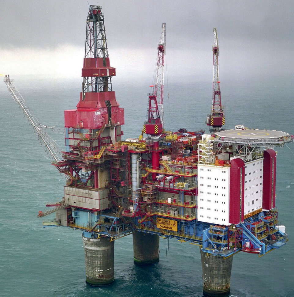
Gullfaks B, Norway. Photo: Courtesy of Statoil.
