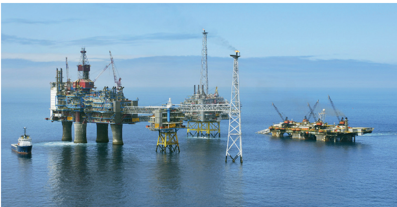
Fire water and seawater lift pumps at Sleipner field. Photo: Courtesy of Statoil.
