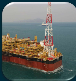
Offshore pumping system
